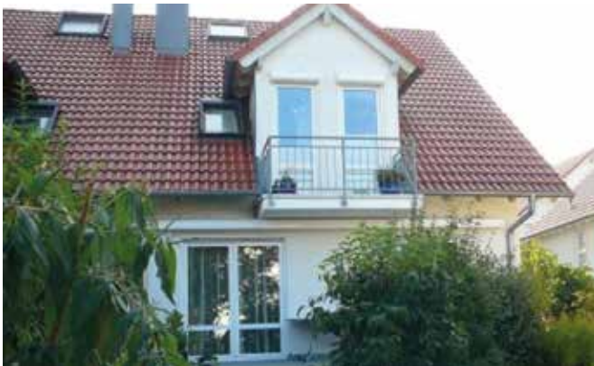
Figure 37: Picture of the house near Stuttgart, Germany.
